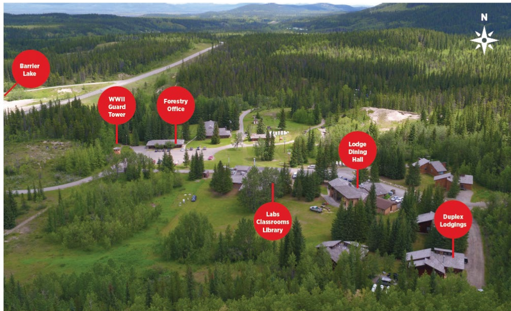
BGI Barrier Lake Field Station
